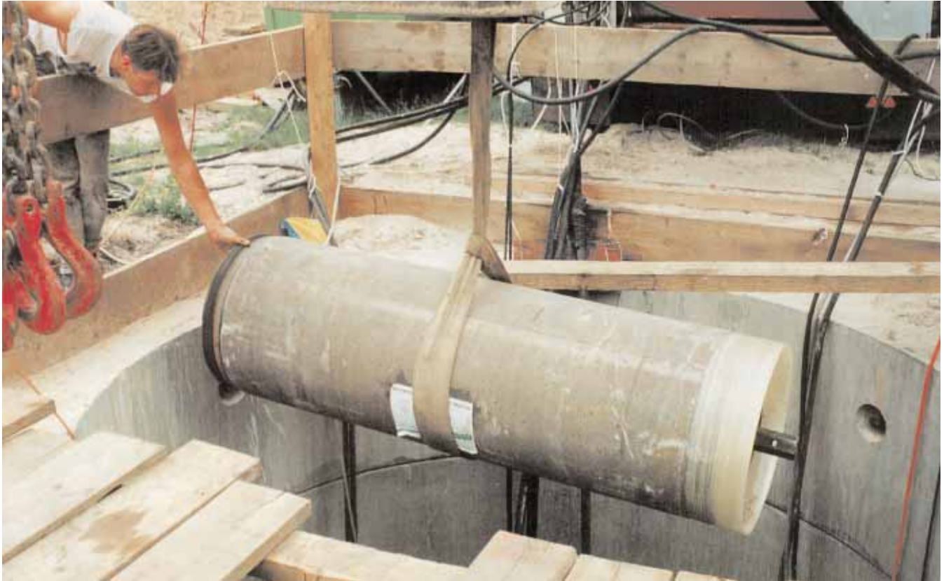
Meyer Polycarbonate pipe being positioned during the Morsbroich Castle pipejacking project.
