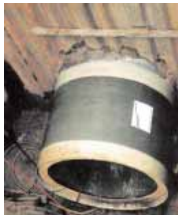
Polycarbonate jacking pipe in the reception shaft
