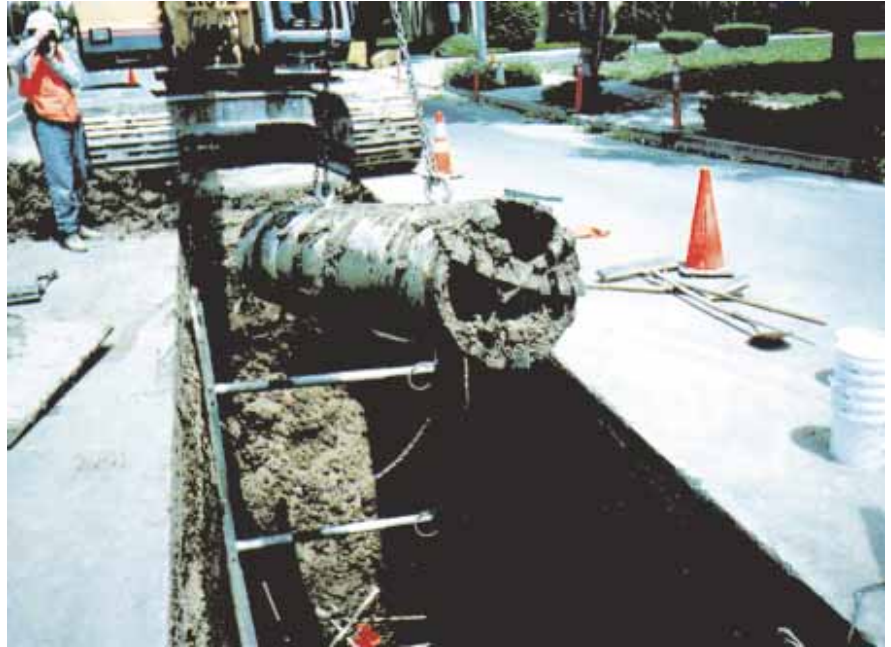
Removing the microtunneller at the end of the drive.
