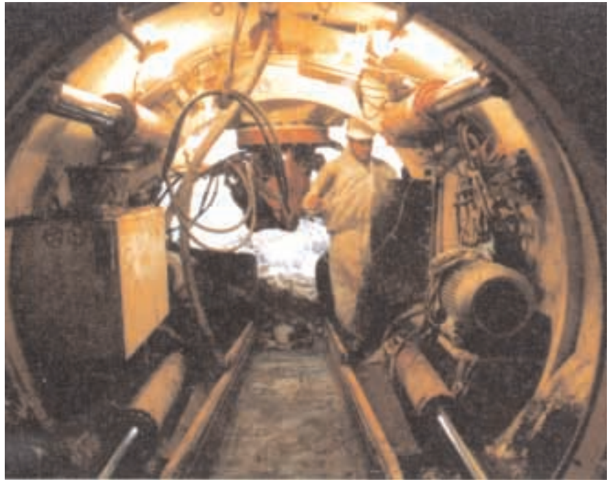
4 Inside view of the cockpit of the driving machine (photo: tis)
