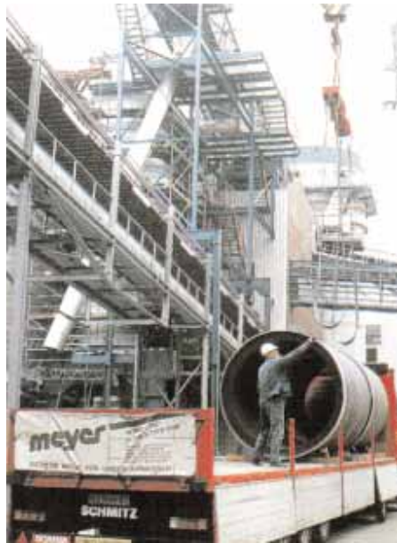
1 Polymer concrete sewer pipes DN 2000 in an industrial plant
