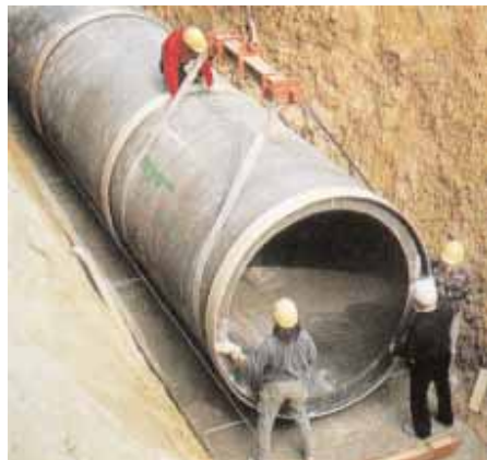
2 Laying of polymer concrete sewer pipes DN 2000
